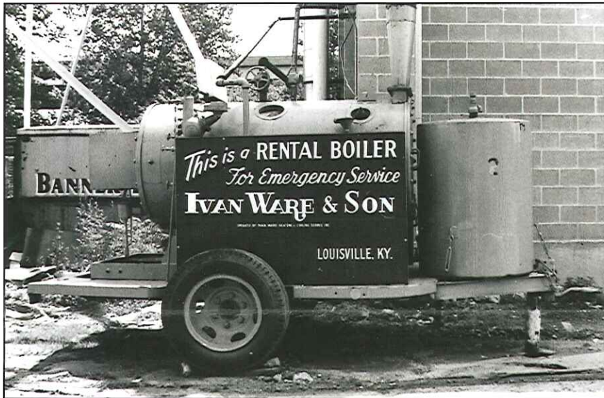
One of Ware's First Rental Boilers
